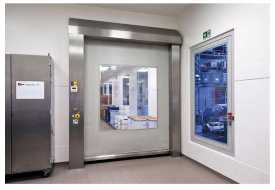
DMF can supply and install specialised high speed doors, designed and constructed to suit highly clinical applications subjected to intense air pressure differences with minimal air loss. The Efaflex SRT CR range can satisfy down to ISO Class 5, and is
