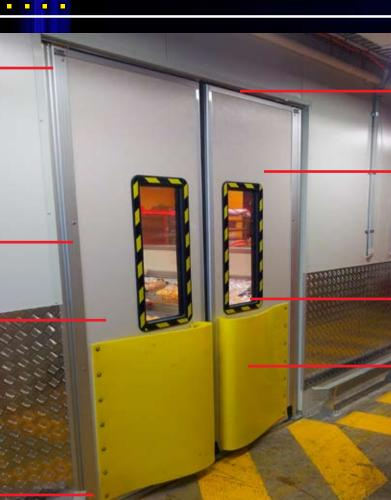
Perimeter aluminium protection, with integrated rubber seals
